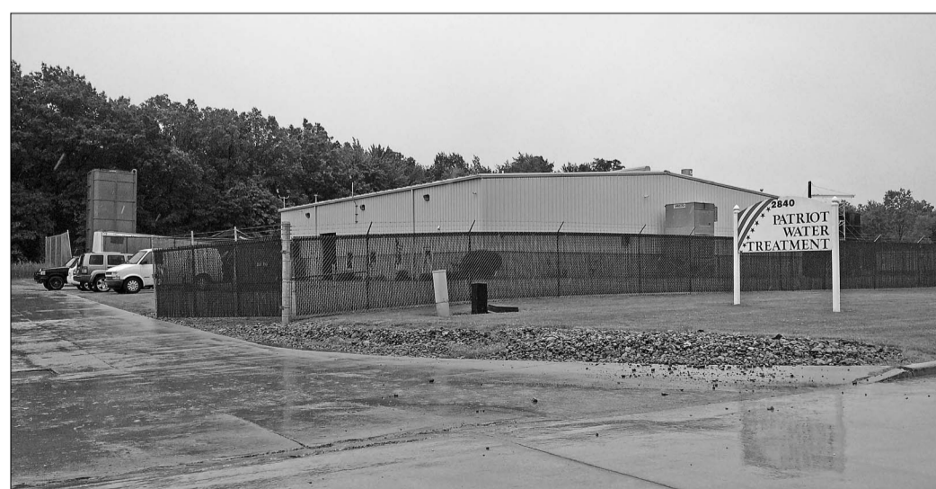
Patriot Water Treatment operates this commercial wastewater treatment plant on Sferra Drive in Warren, and has been identified by the city and other agencies as the source of odors experienced by residents and businesses. The company has told the city that it will address the problem.
