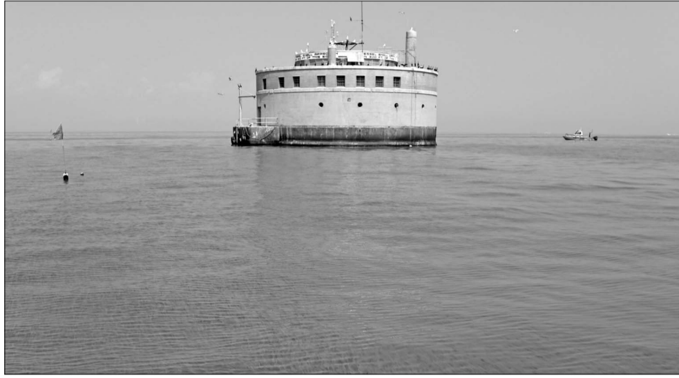
The city of Toledo water intake crib is surrounded by algae in Lake Erie, off the shore of Curtice, Ohio.
