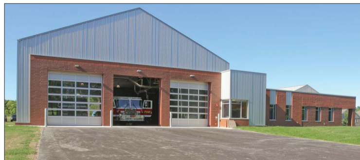
The new Cardinal Joint Fire District station on Herbert Road will decrease response times to areas in the north and west of the district.
