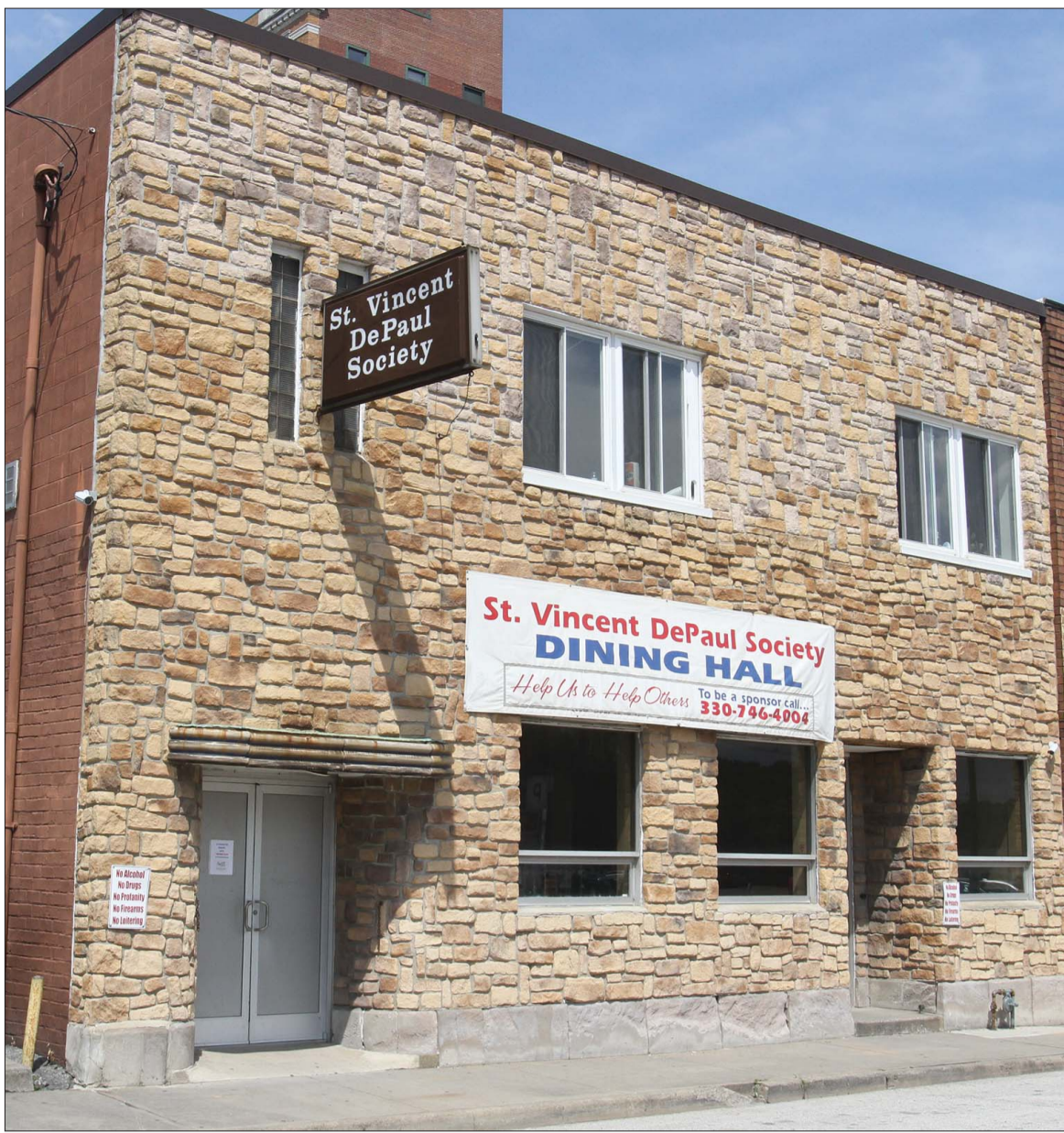
After a ceiling buckled at the St. Vincent DePaul Society building, the Mahoning County Building Inspection Department found it was in violation of the Ohio Building Code.
