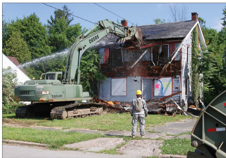
About 40 members of an Army National Guard unit are razing houses on Youngstown's South Side. Among the structures that came down Monday was this vacant one on Clearmount Drive.
