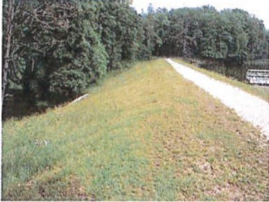
Dam embankment prior to severe flood.
