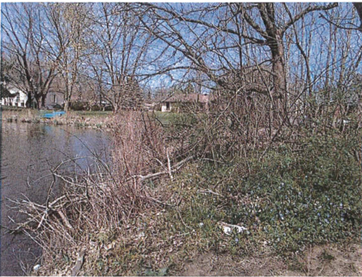
Photograph No. 2: Another view of the upstream slope.
