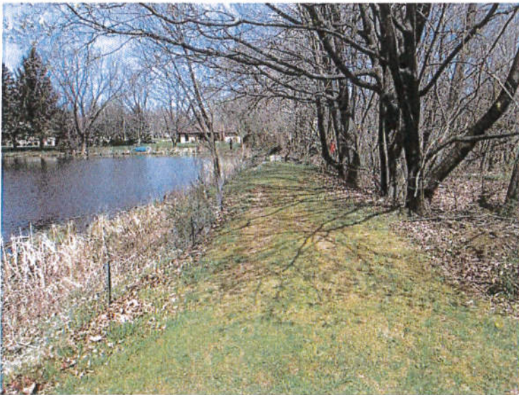
Photograph No. 3: View of the crest from the right abutment.
