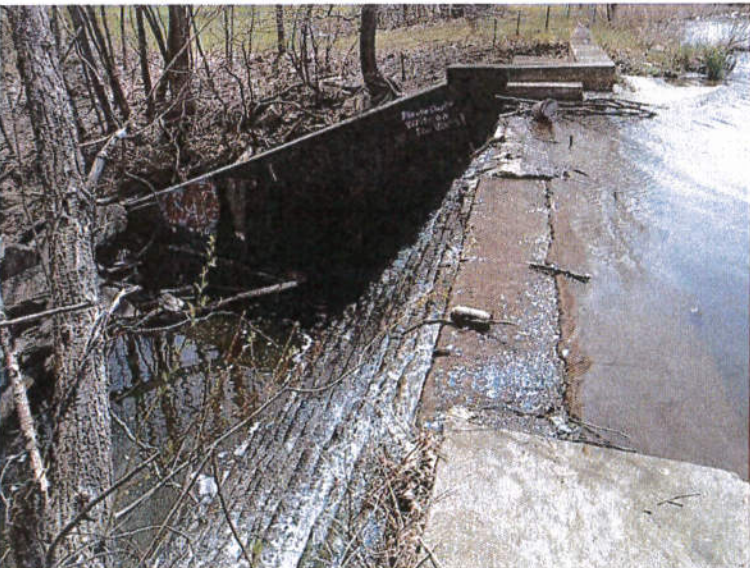
Photograph No. 6: View of the principal spillway weir.
